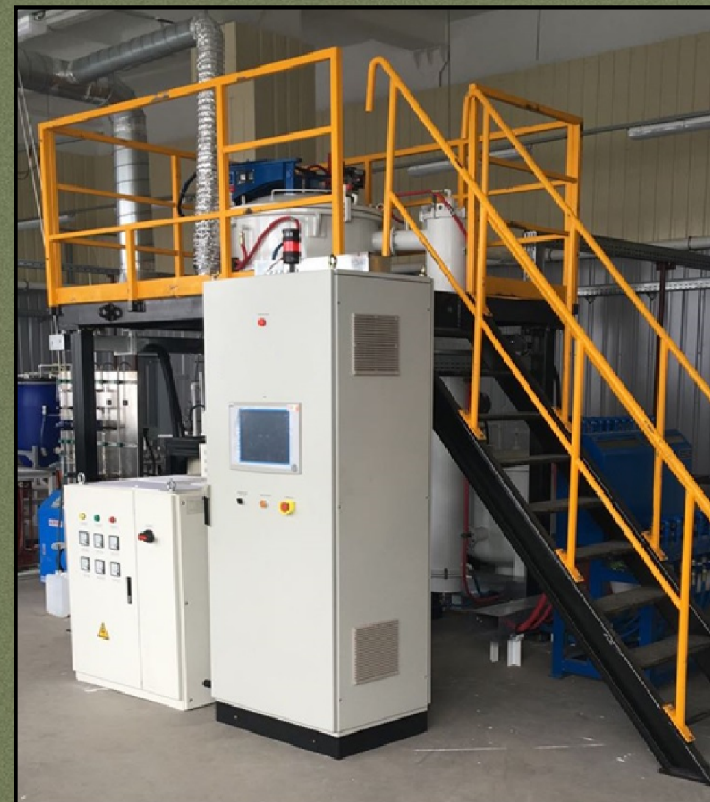
Silicon carbide Deposition Plant (MTS)
