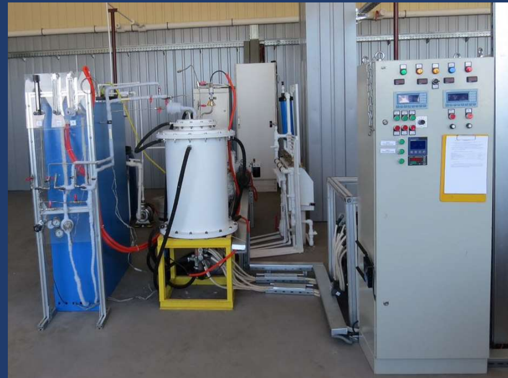
Pyrolytic Boron Nitride Deposition Plant 2.0
